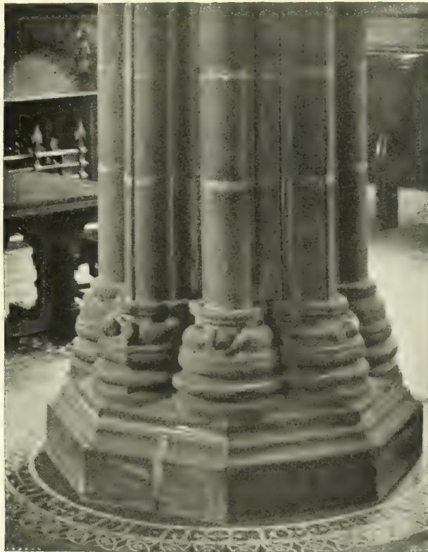
Base of Column in Sacristy.
